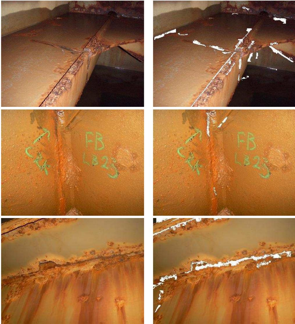
Figure 3: (1st column) Test images and (2nd column) detected cracks
